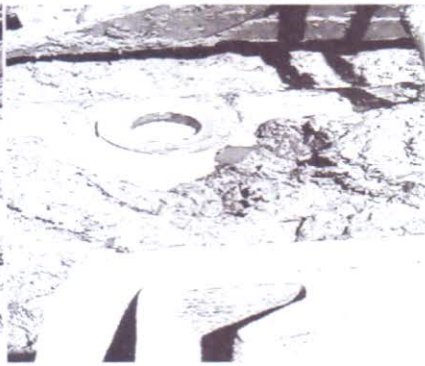
Picture showing point with cofferdam. Picture showing 6 " flange welded on the pipeline.
